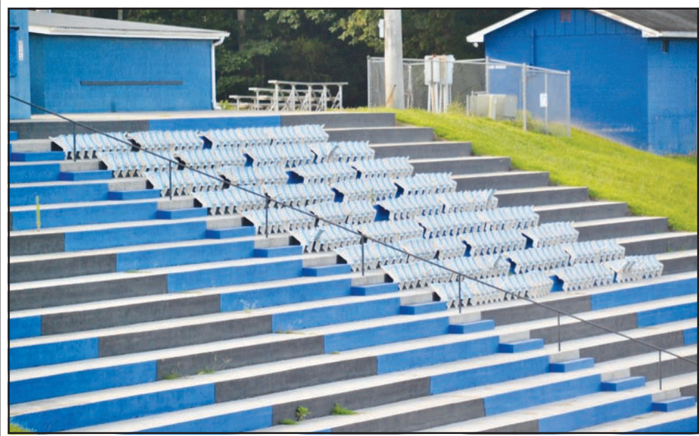
Frank McClure Memorial Stadium is getting upgraded seating on the stadium bleachers. Photo by Chad Stack
